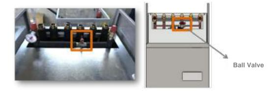
The valve must be opened for the filling of the hydraulic circuit (DHW circuit and central heating&cooling). Before putting the heat pump into operation, check that the hydraulic circuit is full and properly purged. If these two requirements are met, the valve must be closed.
