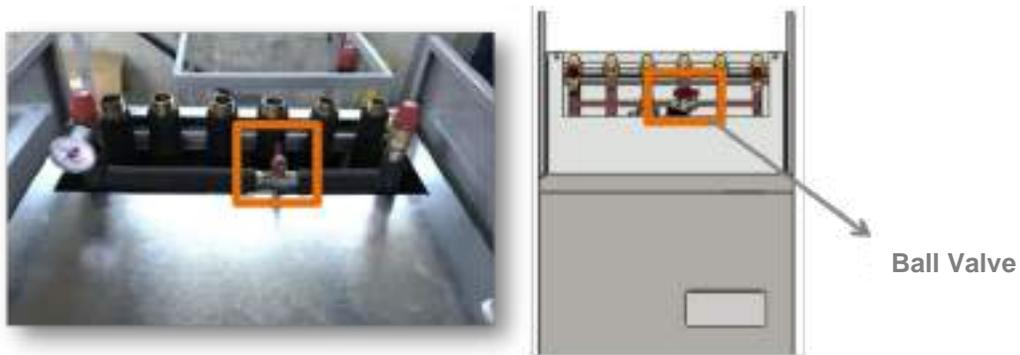
The valve must be opened for the filling of the hydraulic circuit (DHW circuit and central heating&cooling). Before putting the heat pump into operation, check that the hydraulic circuit is full and properly purged. If these two requirements are met, the valve must be closed.
